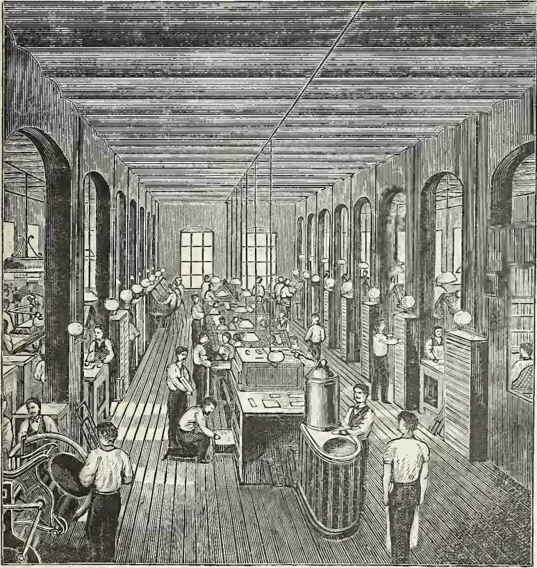
PRINTING DEPARTMENT—Job Room.
